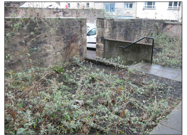
3. Existing Rear Yard.
